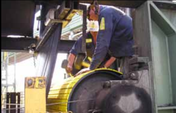
Drum Lagging on site
